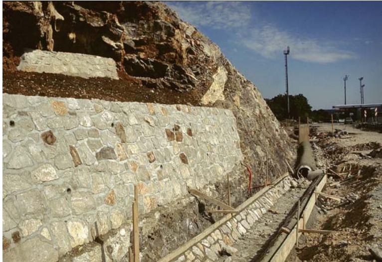
Fig. 2: Construction of an impermeable roadbed through a cutting where a breached cave has been walled off.
